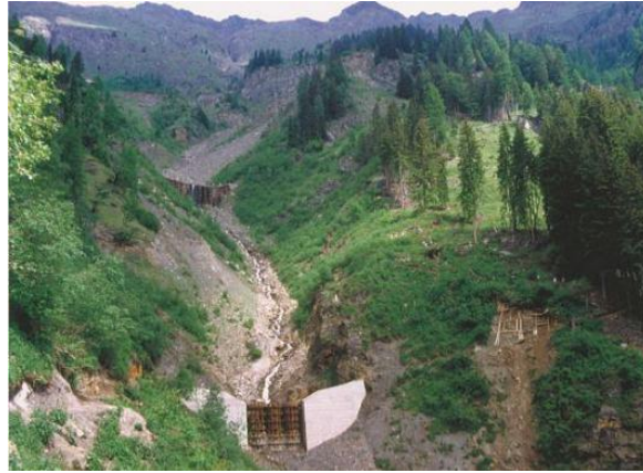
Permanent check dam, Austria
