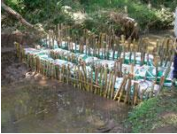
Small check dam, Thailand
