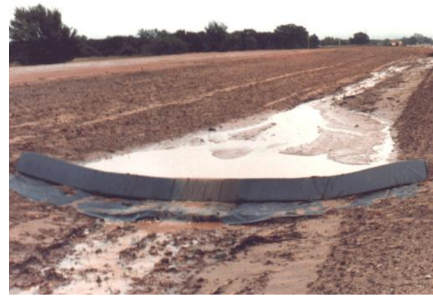
Temporary check dam
